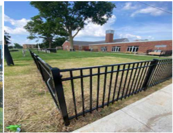
New fencing for playground area.
